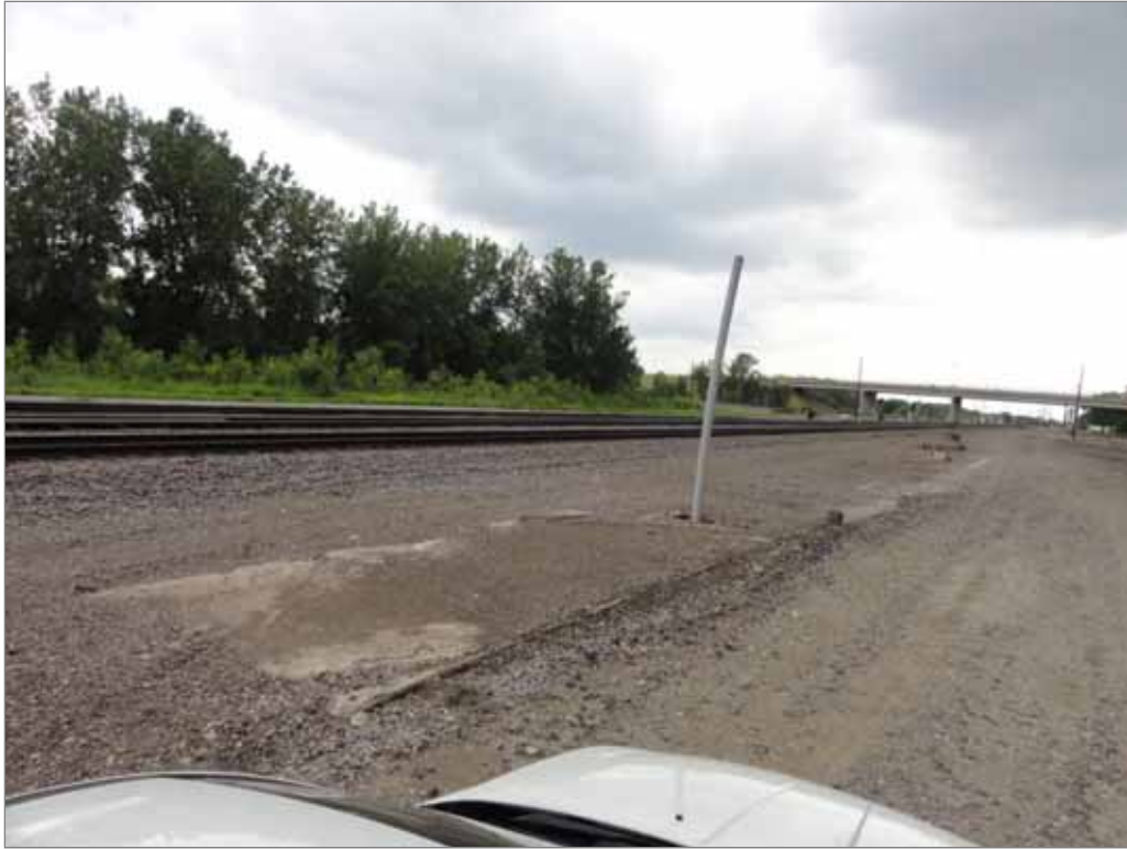
Photo 1: Concrete Slab Foundation
